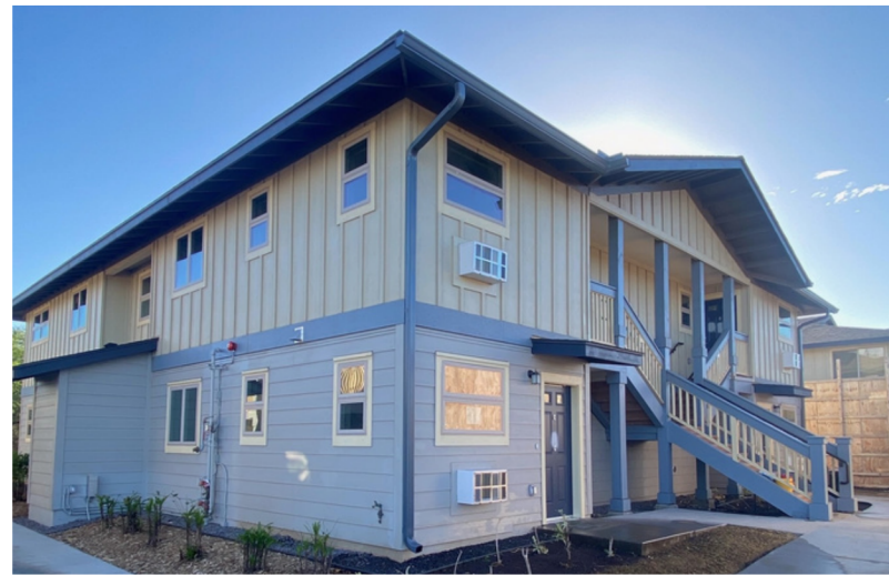
Units at Waikoloa Family Affordable are ready for occupancy. Courtesy photo
