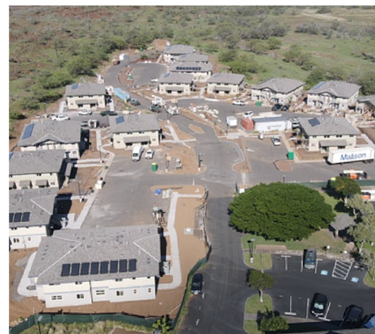
Waikoloa Family Affordable is seen this spring as construction wrapped up on the affordable rental project in South Kohala. Courtesy photos
