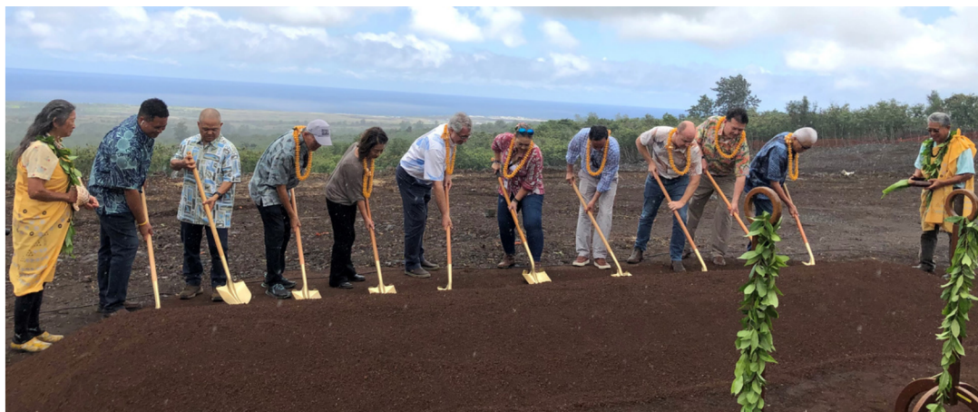
Dignitaries break ground for the Kaloko Affordable Housing Project during a ceremony Friday, April 28, 2023, in Kailua-Kona. Photos Courtesy of County of Hawai'i
